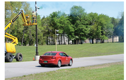
The one-day test evaluated infrastructure-to-infrastructure and infrastructure-to-vehicle communications.
